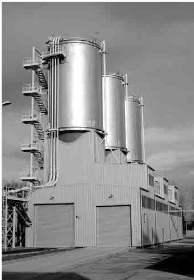
**Pic. 3. Installation of dry ash collection**
